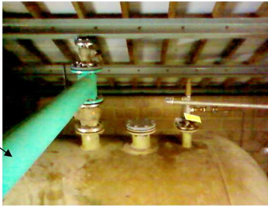
**Figure 7 Photo of Balance tube by courtesy of Ian Currie of Quantum Engineering**
